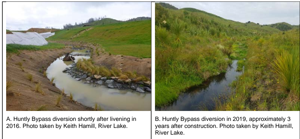
Figure K6 Examples of permanent stream diversion channels created during highway construction projects.
