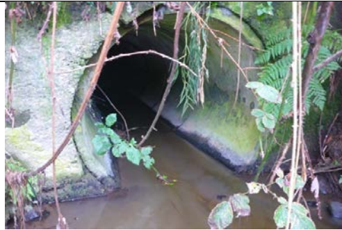
Stream 2 culvert beneath SH1 (12 April 2021)
