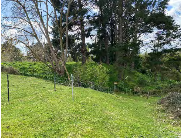
Toe of landfill, view north
