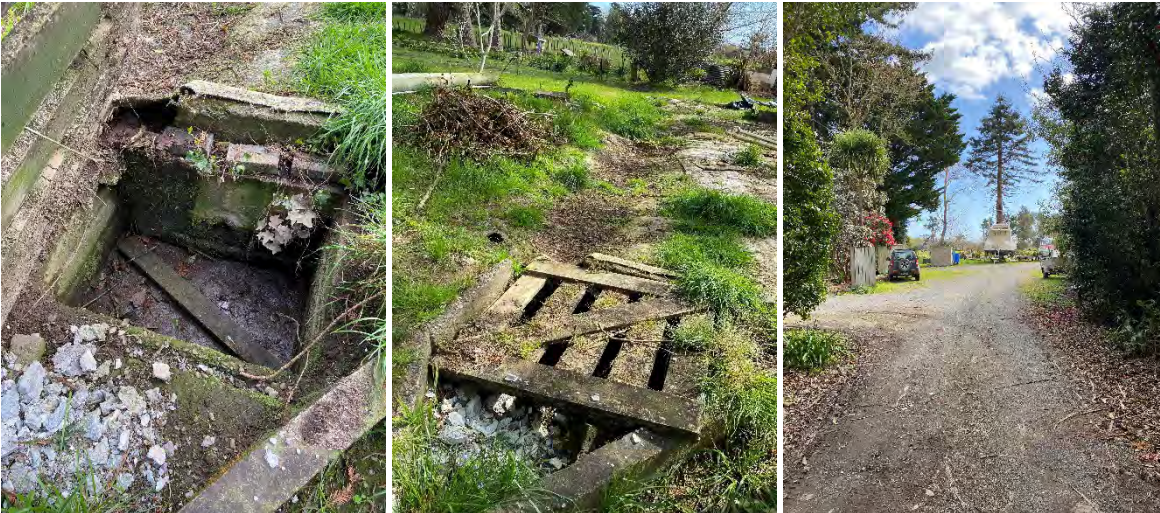
Figure 13 Sump and soak away area at 380-386 Arapaepae Road (HAIL ID 10)
