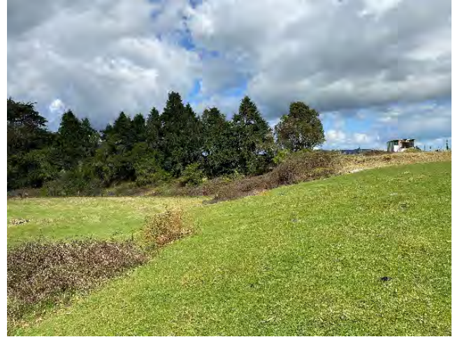
Toe of landfill, view south
