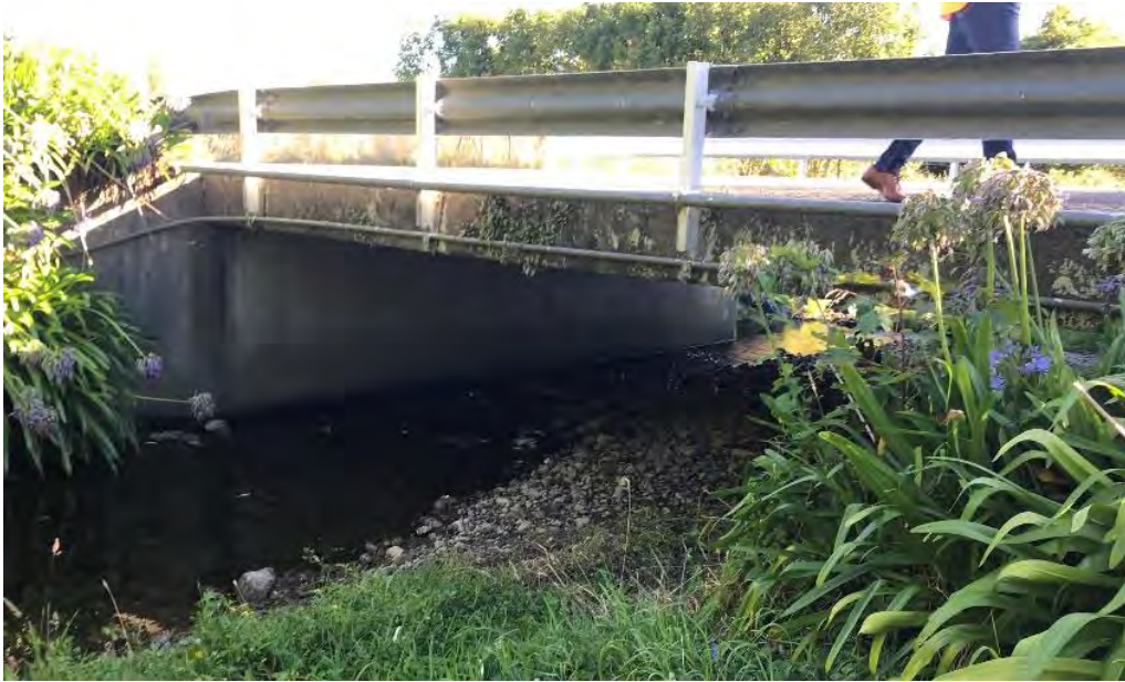
South_Manakau_rd DS Inside Bridge
