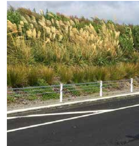
Mackays to Peka Peka Expressway [Natural Habitats https://www.naturalhabitats.co.nz/our-projects/mackays-to-peka-peka/ ]
