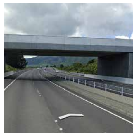
Ngarara Bridge, Peka-peka to Ōtaki. Highway under local road Ref: Google Street View
