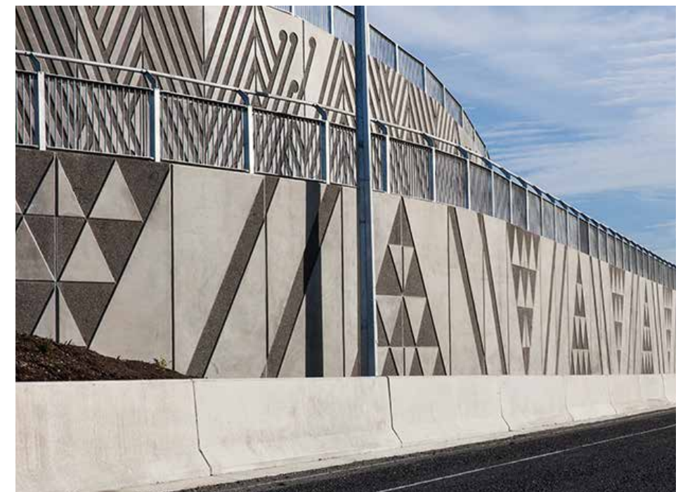
Te Kakakura Retaining Wall [ https://www.boffamiskell.co.nz/news-and-insights/article.php?v=te-kakakura-retaining-wall ]
