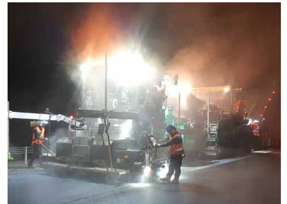
Low-noise surface being installed, Christchurch Northern Corridor [Altissimo Consulting]
