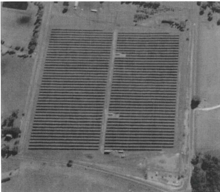
Melbourne Airport solar farm. Note the absence of screening.
